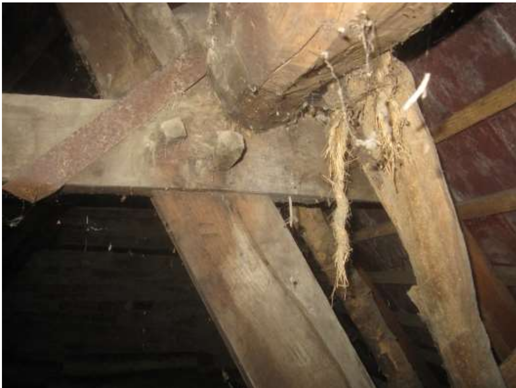
Detail of lap-jointed collar to truss T1
