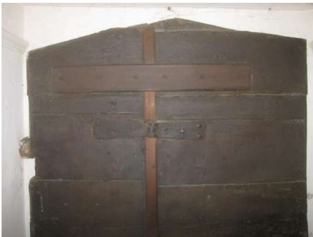
Rear face of door to No 6, with centre-folding hinge
